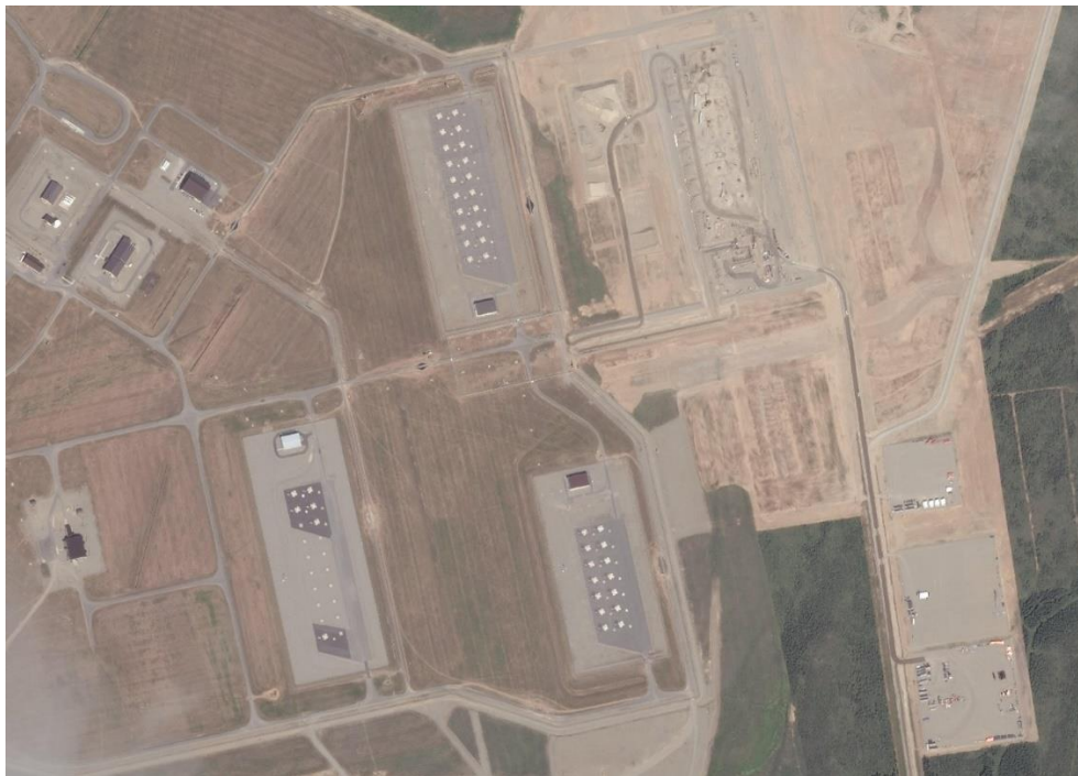
This satellite image of the Fort Greely, Alaska missile defence base shows three fields of ground-based missile interceptor silos (accommodating a total of 40 operational interceptors), with a fourth missile field under construction (upper right). That will bring the strategic missile defence system to 60 Alaskan interceptors plus four in California. (Image by SecureWatch/Maxar Technologies)
