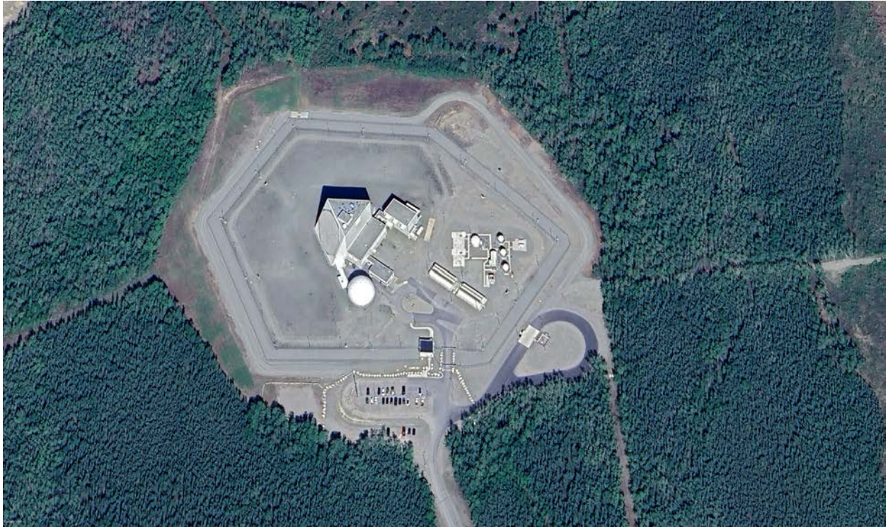
Fig. 9: Alaska's Clear Space Force Station operates a Long Range Discrimination Radar designed to scan polar and north Pacific regions as part of the strategic missile defence system. Google Earth
